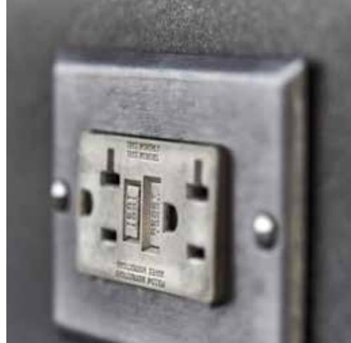
Ground Fault Circuit Interrupter (GFCI) outlets should be used in any area where water and electricity may come into contact
